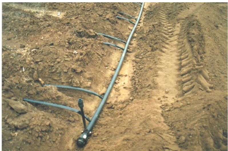
Flushing Manifold prior to burial.
