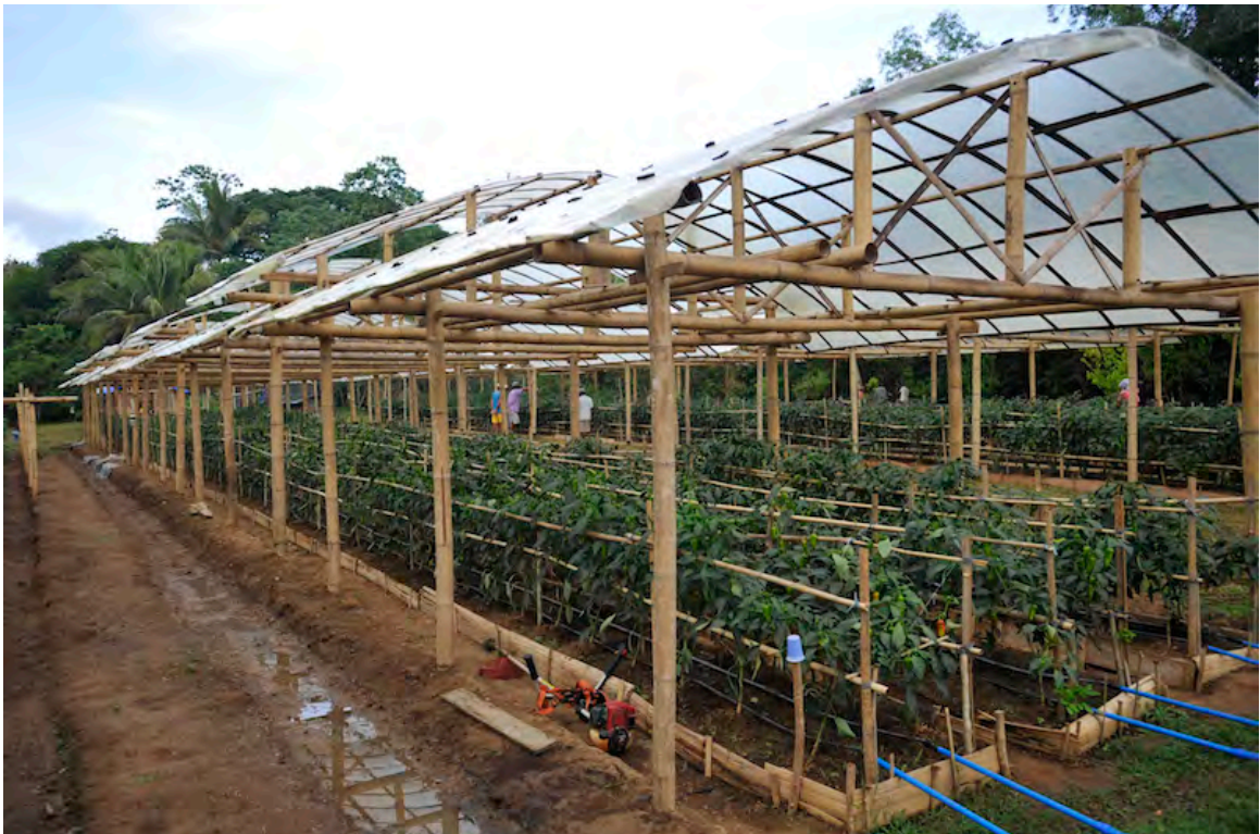
Photo 3. Curved roof design (NSW DPI)
