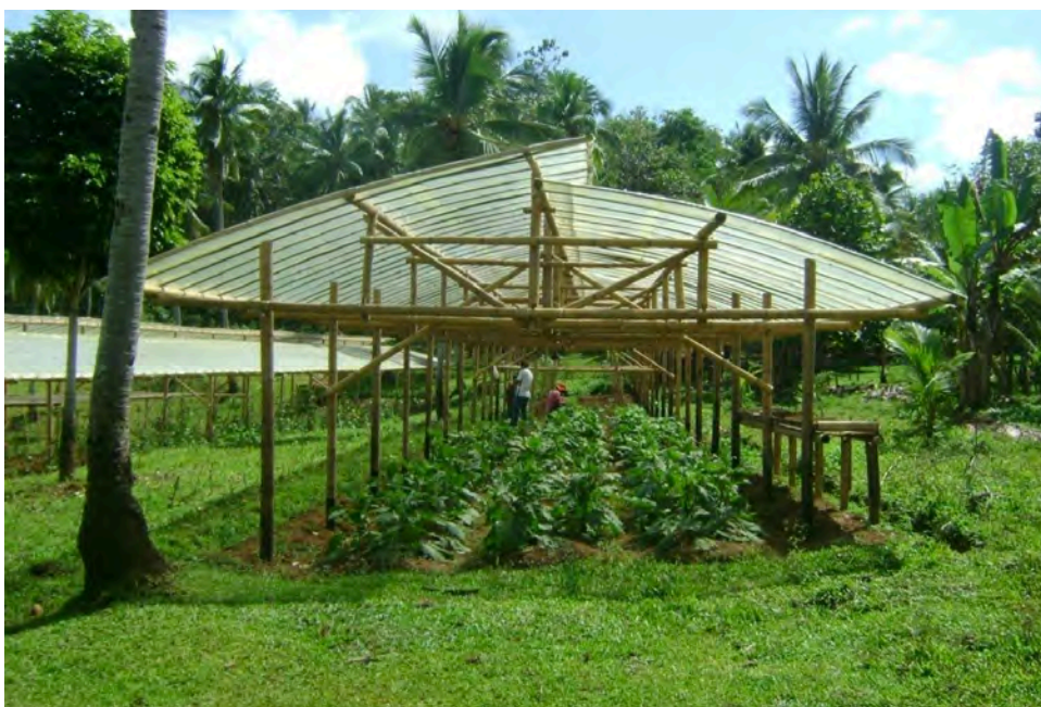
Photo 5. Modified curved roof system.
