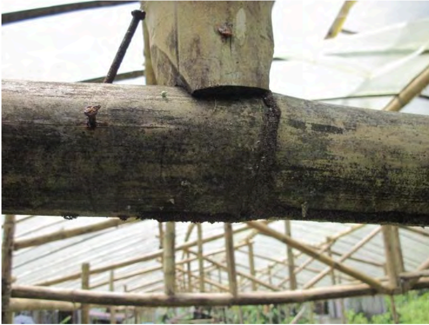
Photo 10 Termites attacking the bamboo
