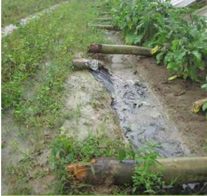
Photo 8. Rotten bamboo posts
