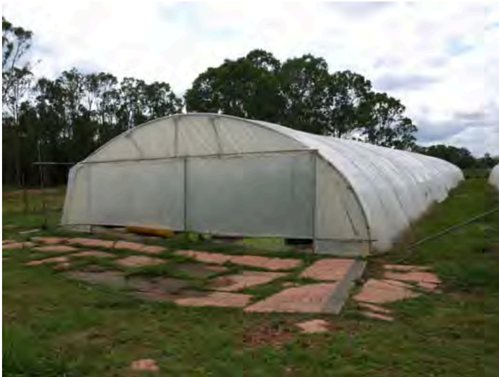
Photo 14. A typical tunnel house
