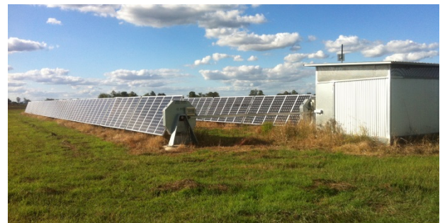
Figure 20: Panel orientation at 12pm and 3.30pm in late April – effect of the tracking system
