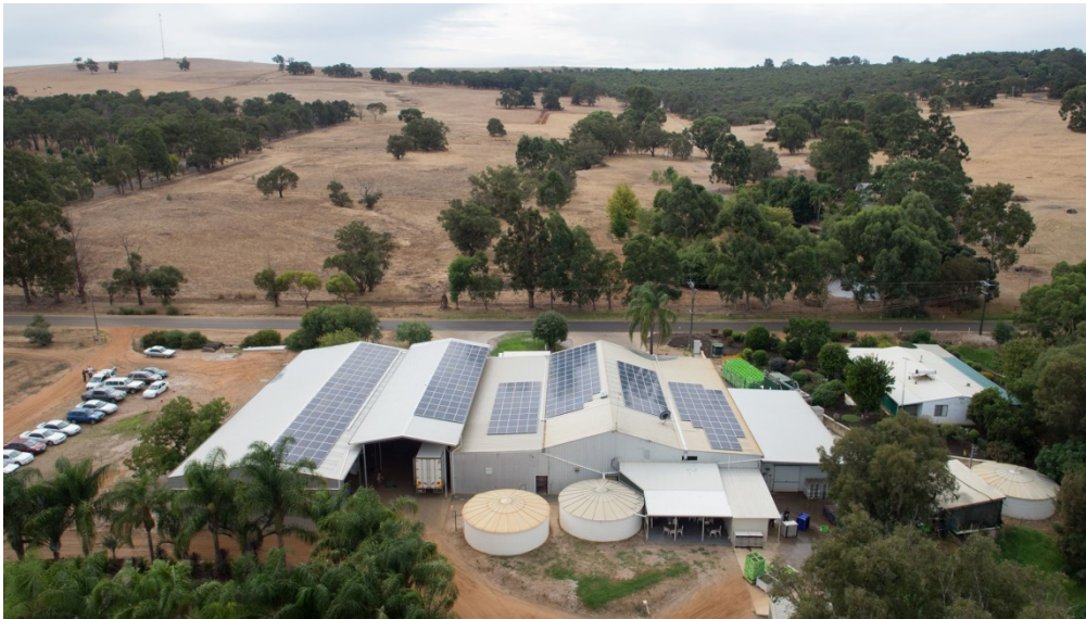
Figure 12: Loose Leaf Lettuce Company 100kW rooftop solar installation
