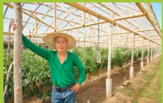
Boie Gerona with the structure he designed to withstand strong wind and rain.
