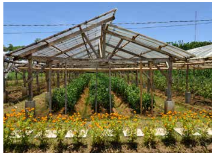
House-type structures can be made with a curved roof (top), or flat roof with a ventilation gap (bottom).
