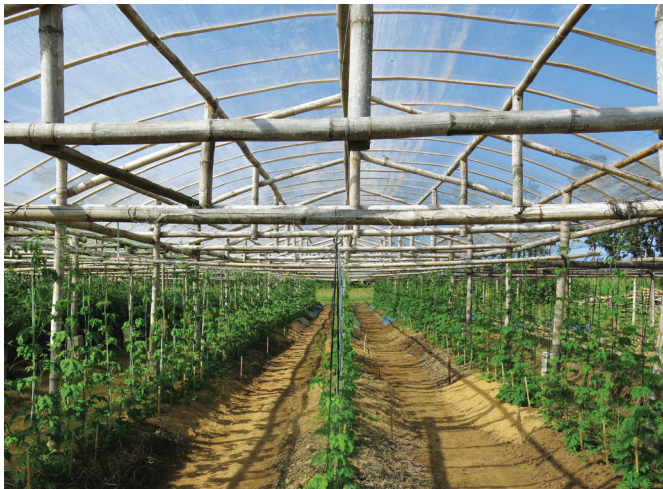
Protected cropping structure showing trellising.
