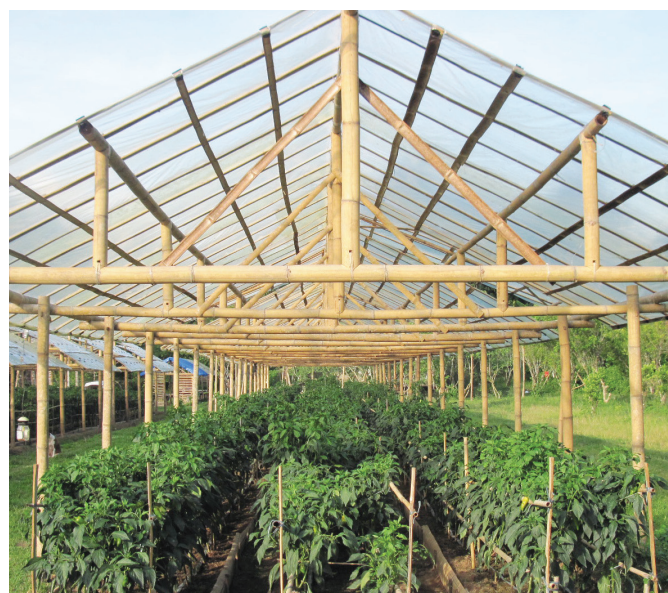
Sweet pepper under a house-type protective structure made from bamboo
