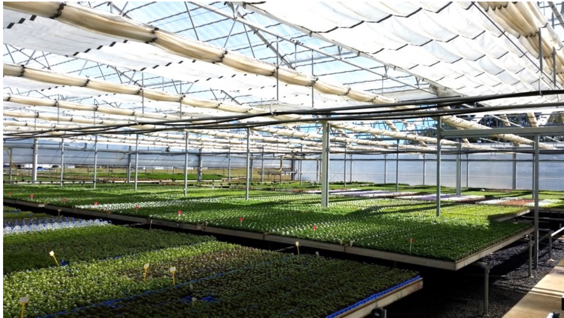
Figure 1. A retractable roof Cravo® house used to grow vegetable seedlings in Gatton, Qld.
