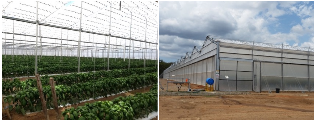
Figure 6. The retractable roof Cravo ® house installed by Young Sang & Co. in Bundaberg.
