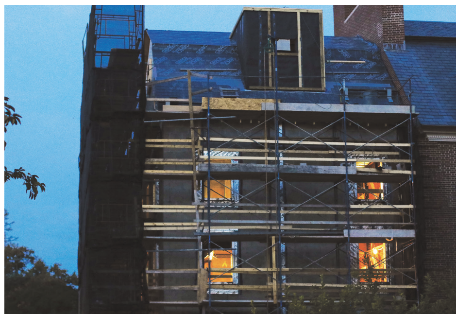
Wentworth Hall will be under construction for the next year.
