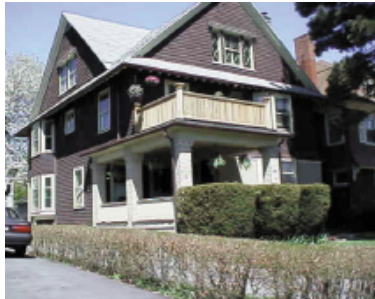
57/59 Calumet - Spring of 1999. New 2nd floor railing, but prior to new roof, new cedar shake and paint which was completed in 2002
