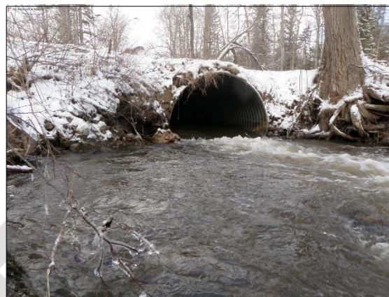
Upgraded culverts can mitigate flooding problems by increasing the flow capacity of streams as they pass under roadways.
