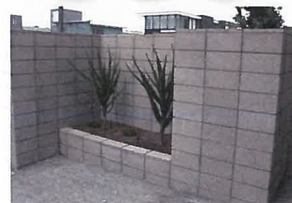
REFERENCE IMAGE CMU STACKED BOND WALL
