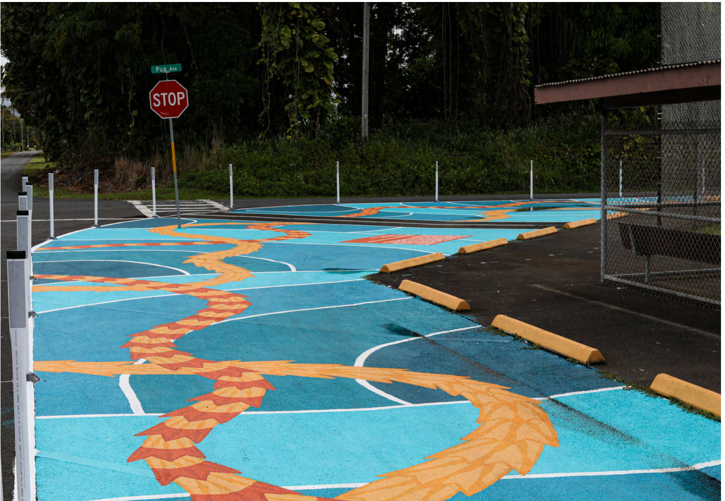
An example of quick-build curb extensions and pedestrian/bike path in Keaukaha, Hawai'i Island. Source: Lanihuli Kanahela, 'A'a Media
