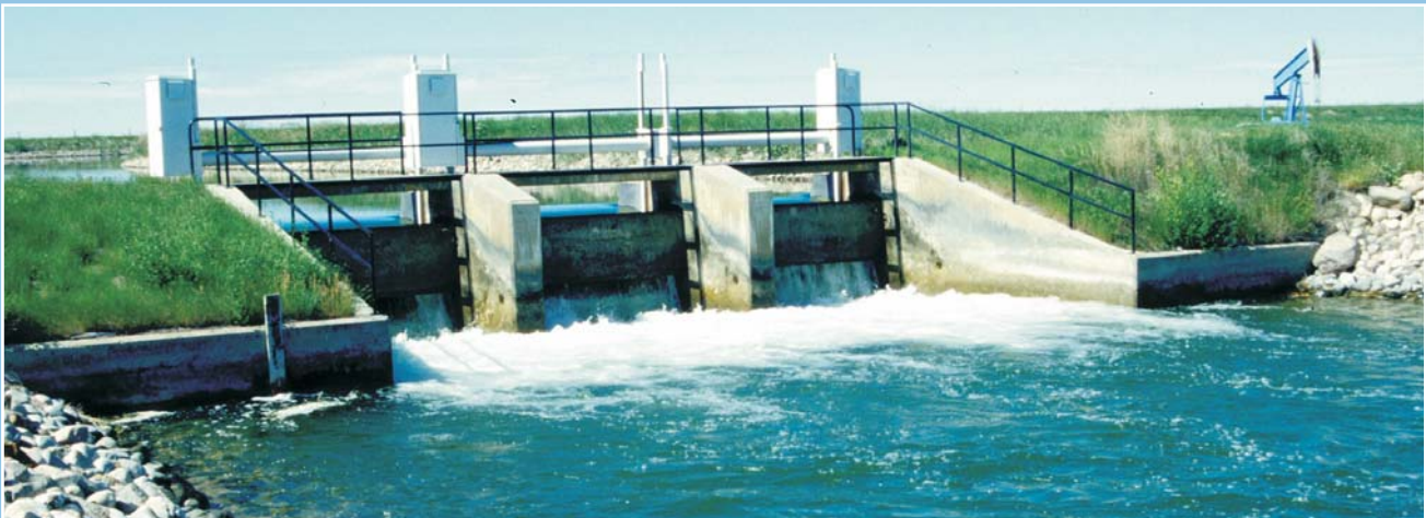
Control structure on BRID canal – AAFRD
