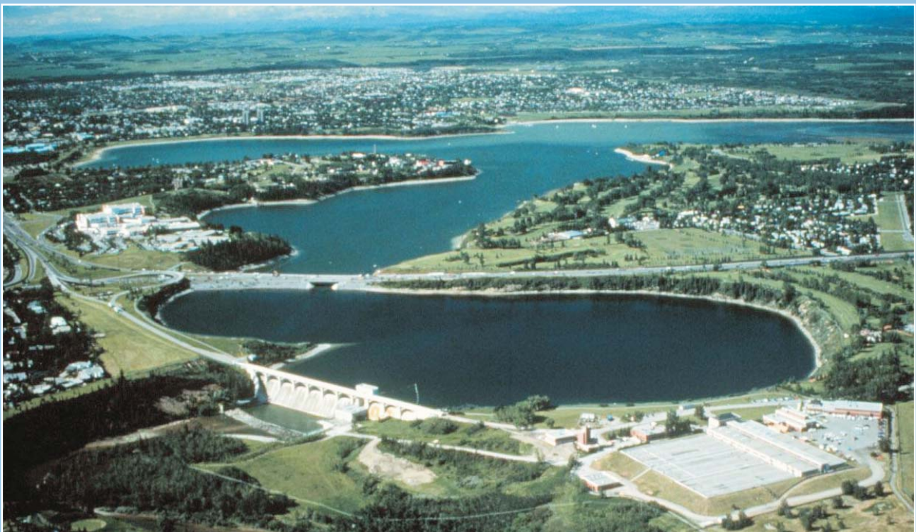
Glenmore Reservoir and water treatment plant – B.Morin
