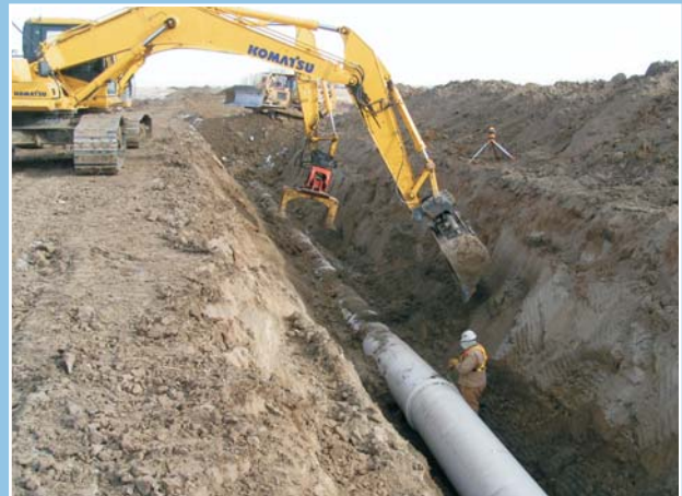
Irrigation pipeline installation in the EID – AAFRD
