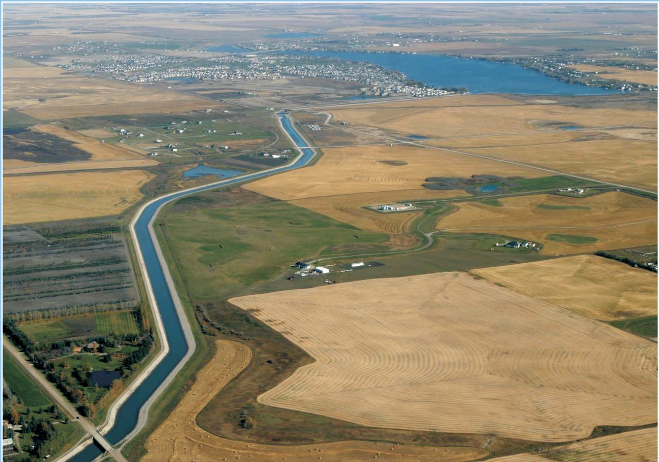
Western Headworks Canal to Chestermere Lake – K.Richardson
