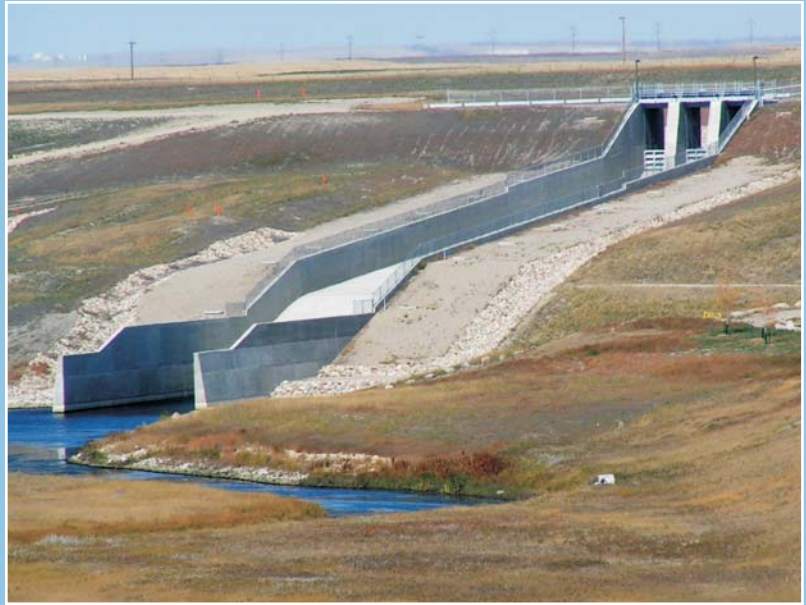
Spillway at Twin Valley Dam – AAFRD
