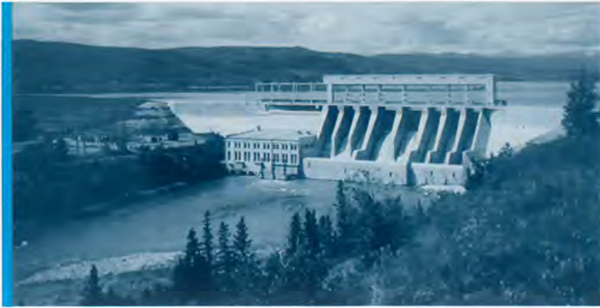
Ghost Hydropower Plant
