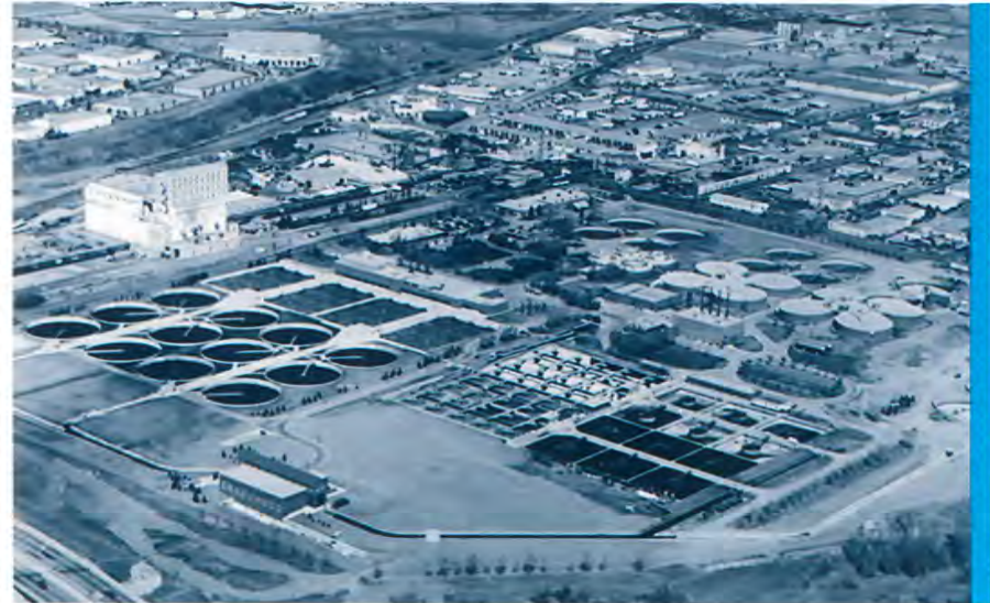
Bonnybrook Wastewater Treatment Plant
