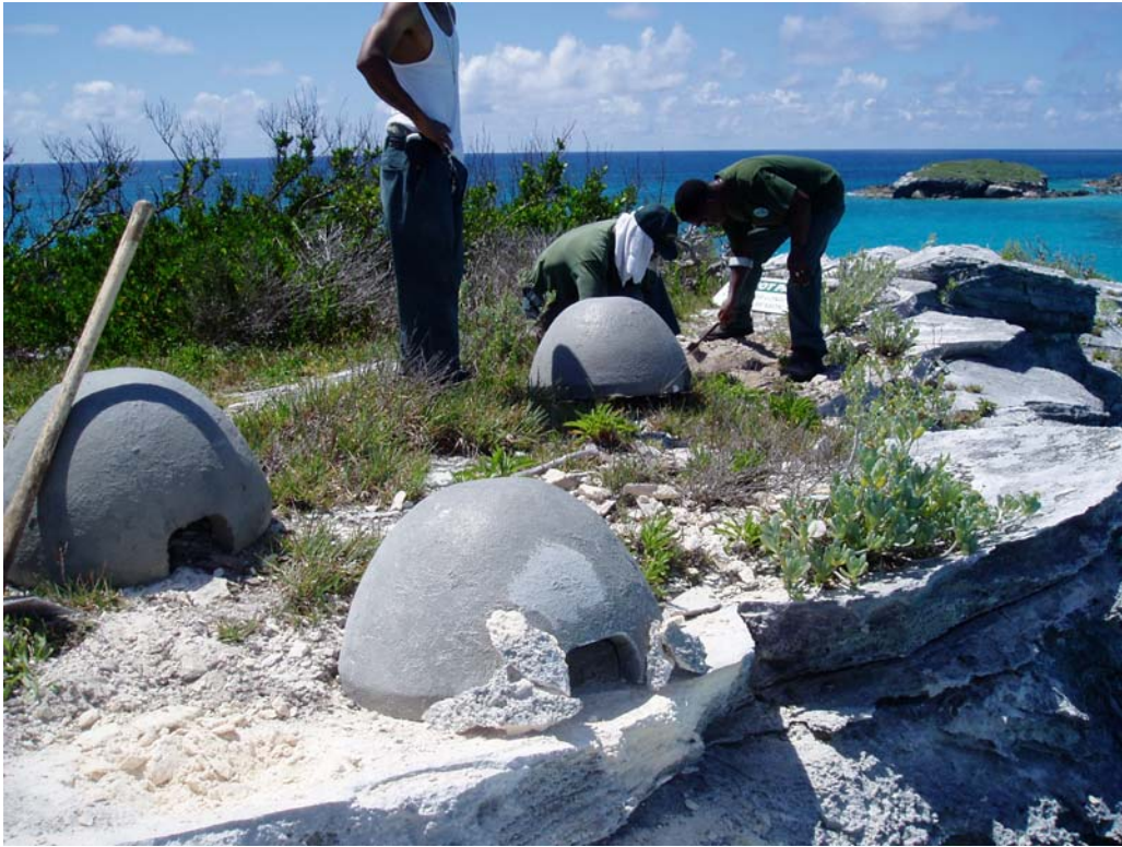
Fig. 8: 'Igloo' nests being cemented to cliff edges by Terrestrial Conservation Crew
