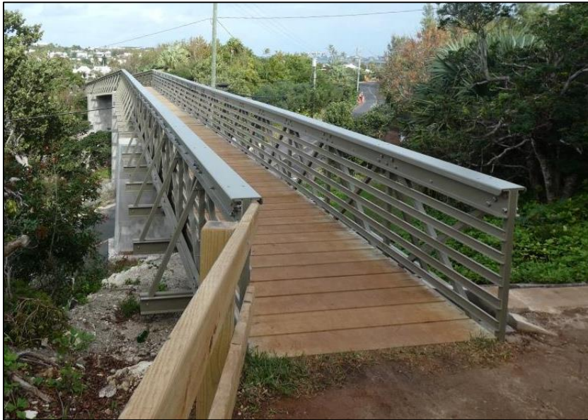
Bridge over North Shore Road at Flatts Railway Trail
