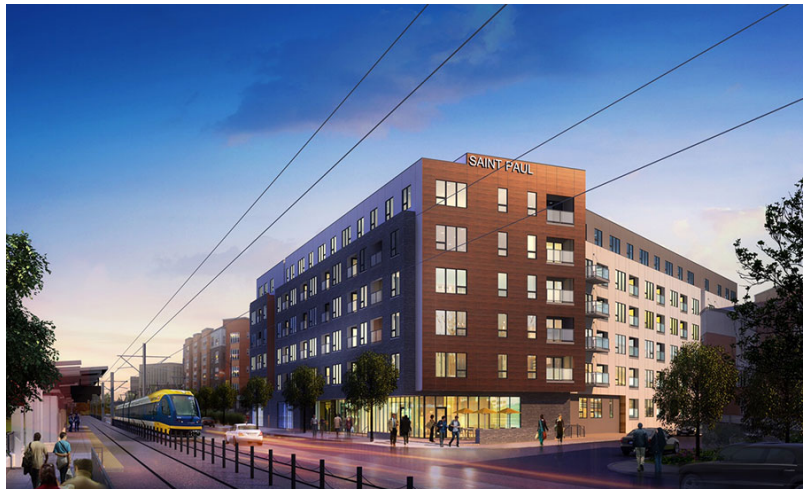
Figure 6. Computer generated rendering of 2700 University emphasizing access to LRT (Source: Flaherty and Collins)
