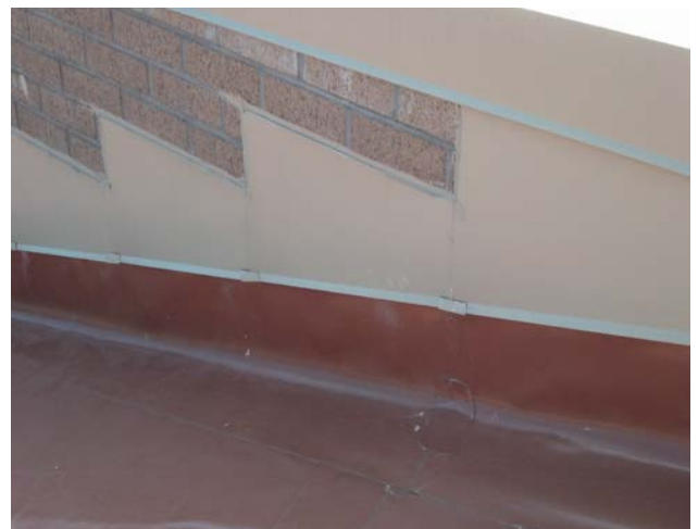
Sidewall Step Flashing – After
