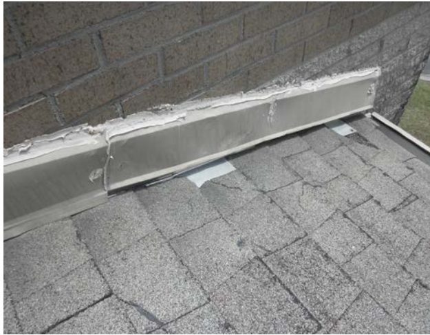
Sidewall Flashing – Before
