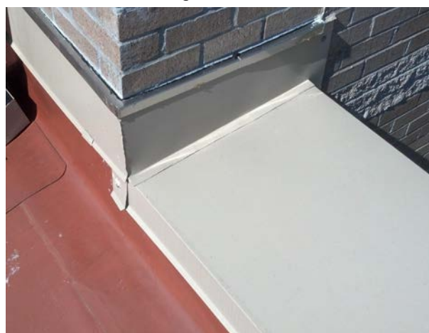
Coping Termination - After
