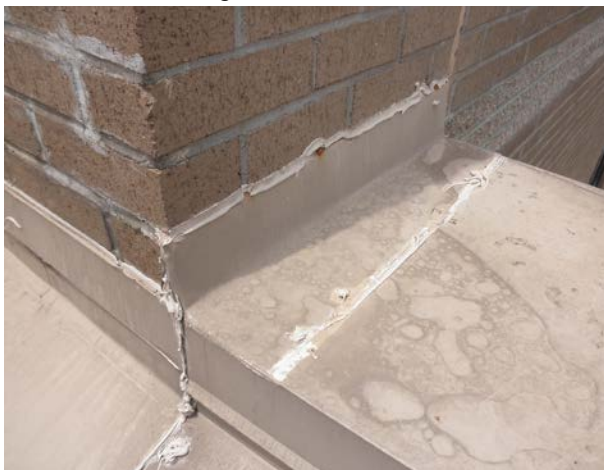
Coping Termination - Before
