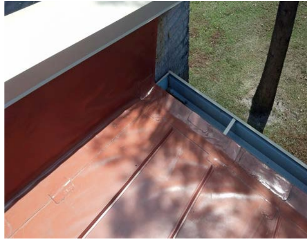
Sidewall Flashing – After
