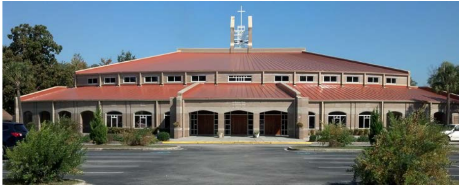
After Photo of Roof
