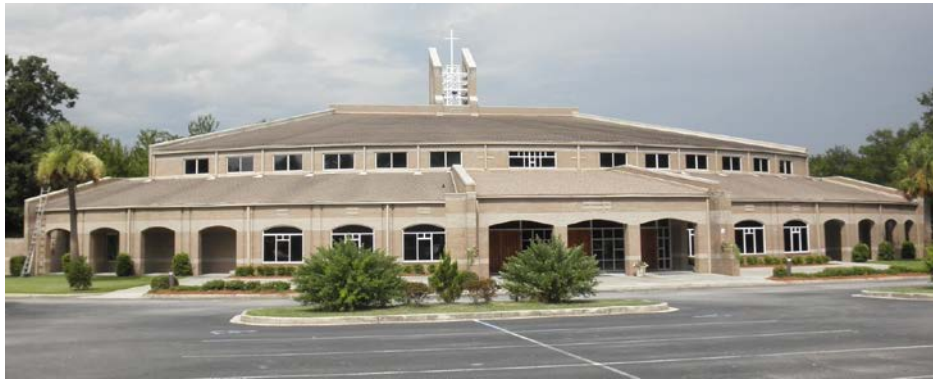
Before Photo of Roof
