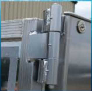
Overslung Sideswing Hinge
