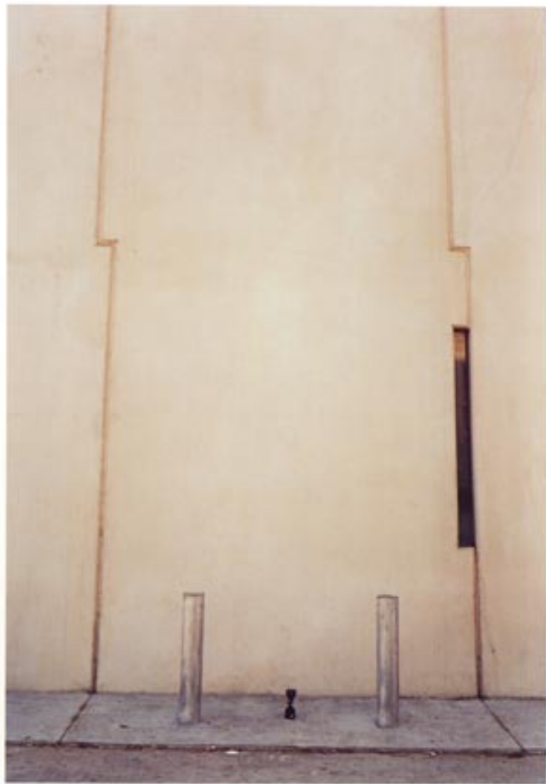
"Because of the confluence of the narrow alleys and the lack of any views, I was really confronted with 'what am I going to do with this large blank wall?'" Hertz recalls. Tilt-up concrete construction offered itself up as the most practical solution.
