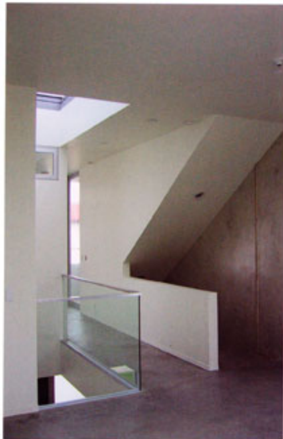
The concrete walls of the interiors are hand-sanded, sealed and waxed, and the floors are burnished. The sound-proofing and thermal properties of the concrete were an added bonus to the clients, who both work from home.
