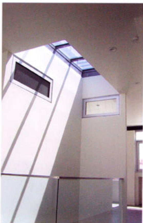
The skylight and atrium below it allow light to penetrate both floors of the front block.
