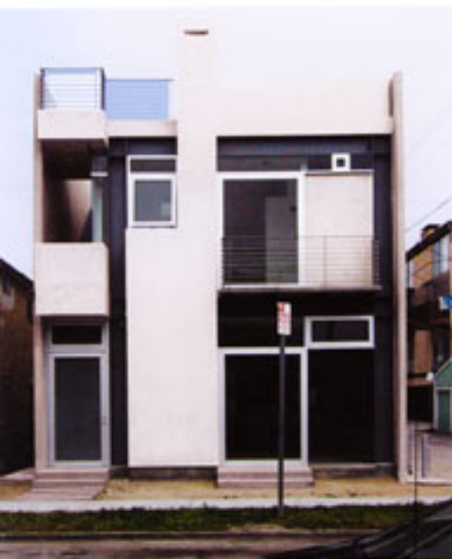
The front elevation. The concrete panels were individually designed to allow for window openings and to articulate the different elements of the façade.
