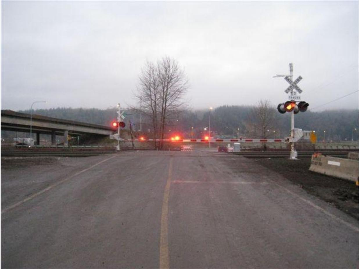
**Figure 4.** Grade crossing now equipped with warning gates and lights.
