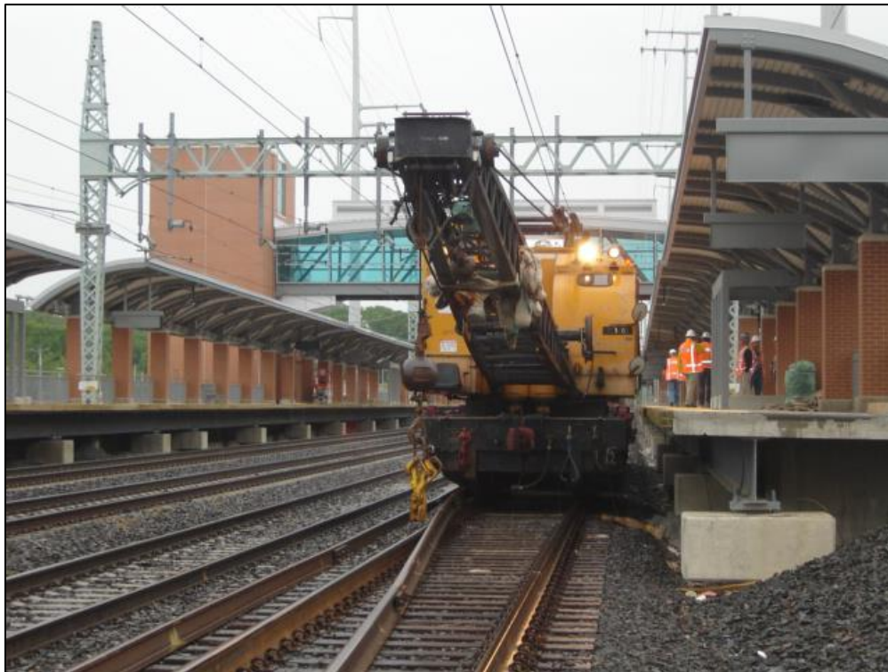
Figure 2. Westward view of work location and crane.
