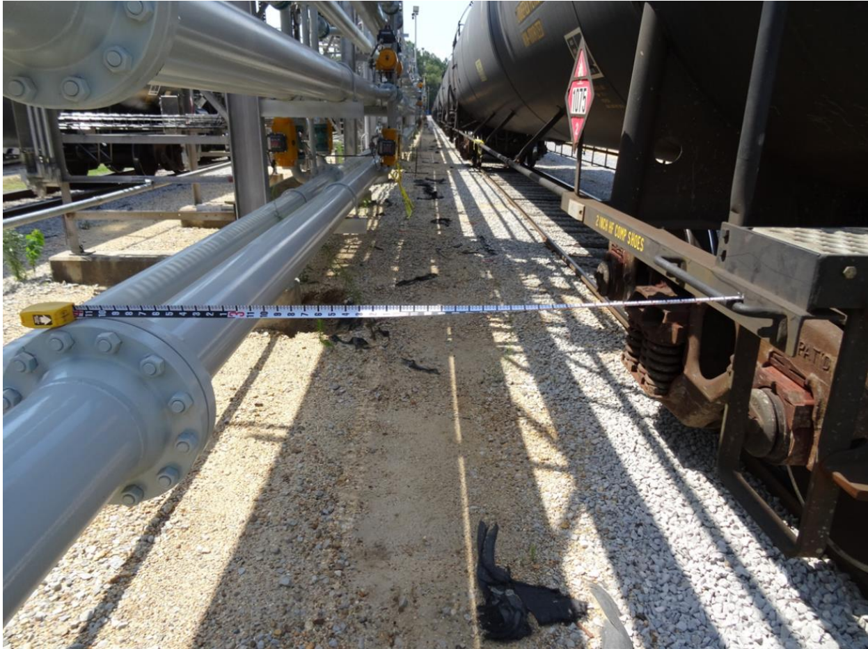
Figure 2. Path between the tank cars and unloading rack in the H 82 gas plant.
