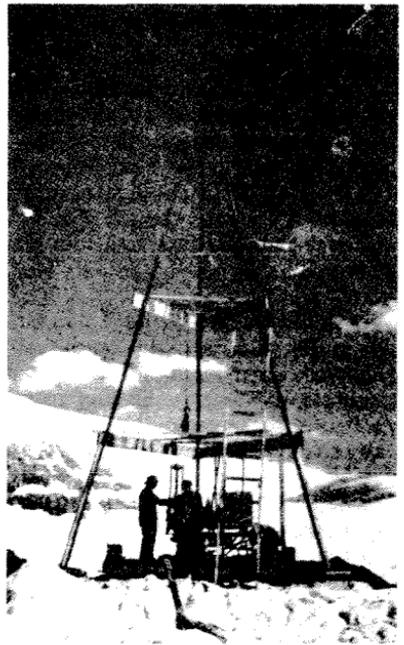
Figure 7. Drill Rig set up at the main camp on upper Taku Glacier, 1950. Cores were obtained to a depth of nearly 300 feet.
