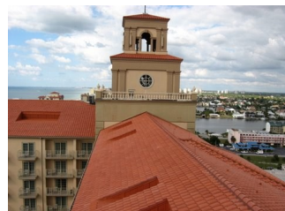
Newly completed tile roof
