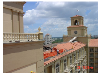
Installation of safety systems
