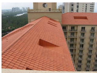
Newly completed tile roof
