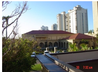
View of low roof areas
