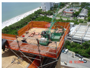
View of roof top hoist area
