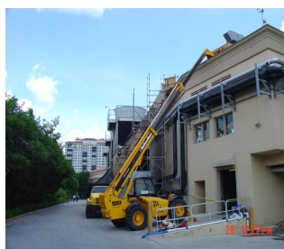
Ground staging area. Used for loading and un-loading roof.
