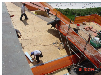
Installing new decking
