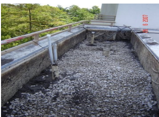
View of planter with shrubs removed
