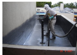
Spray applied Polyurea
