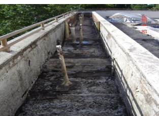
Cleaned and prepped
