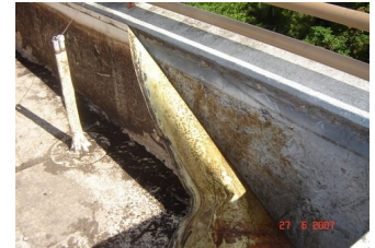
Removing old liner
