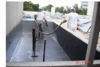
Final touch up of spray liner
