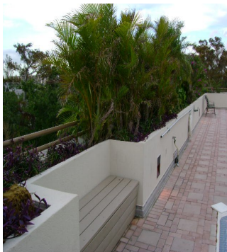
Typical view of pool deck planters on the 4th floor
