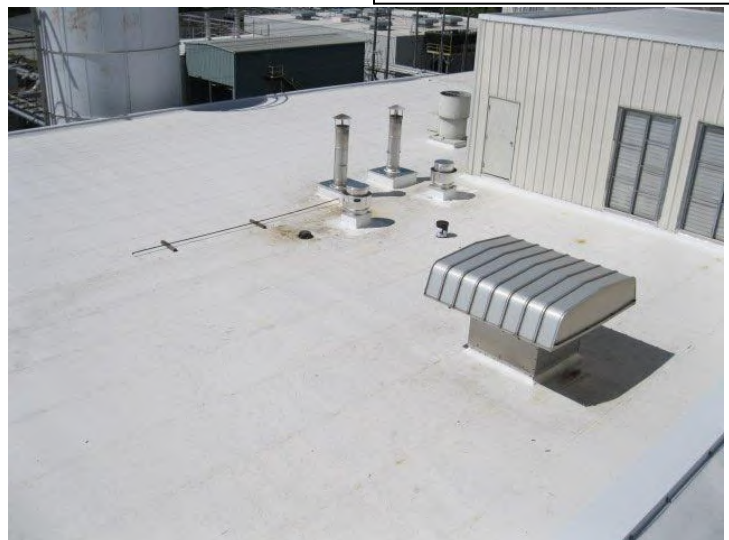
This is a view of the typical detail work.
