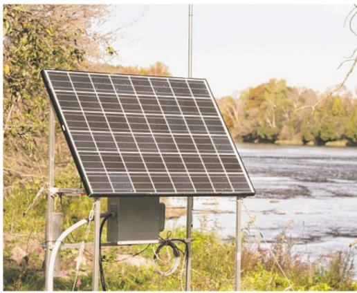
This solar panel powers the Real Time Hydrologic Station located on the Grasse River in Massena, St. Lawrence County. The station, along with 20 others set in and along the Hudson River and other waterways, is part of the Beacon Institute’s River and Estuary Observatory Network. COURTESY PHOTO
