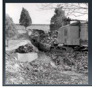
1974, New treatment plant and 36" water line constructed to the Reservoir. In total, there are 36", 20", 14", and 12" water lines on the existing Reservoir site.
