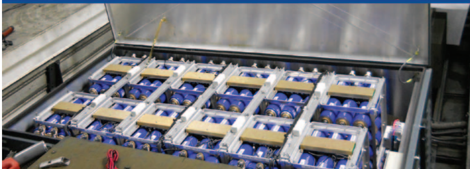
Clockwise from top left: The double layer capacitor enclosure, the power control unit, and the double layer capacitor modules.
