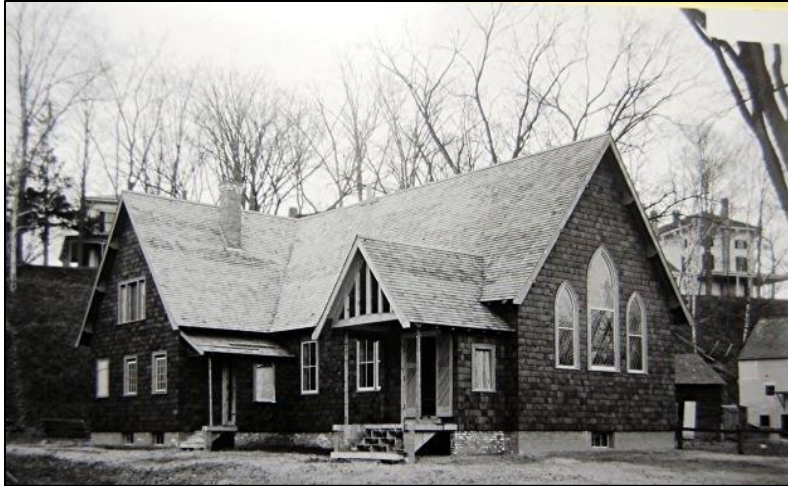
Church of the Epiphany (Episcopal), School Street, Lisbon
