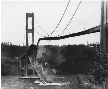
stressors cause the Tacoma Narrows bridge to collapse<sup>26</sup>
