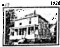
This plain, 2 storey, hip roof house, with an open front veranda, was built in 1926. It is shingled, trimmed by cornerboards, and is intact in its original style.
