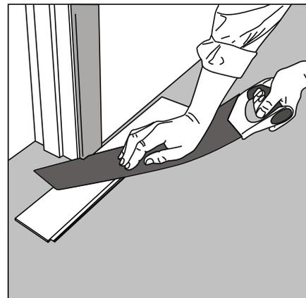
Door mouldings and skirting's: Put a panel (with the decorative side down) next to the door moulding and saw as shown in the figure. Then slide the panel under the moulding.
