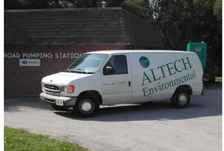
Pumping Station Building
