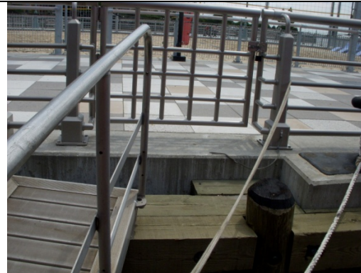
Gangway gate aligns with electrical grounding cord (dark line towards right side of gate aperture) so gangway cannot go there.
