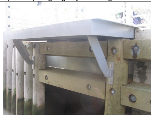
Another view of LILAC cantilevered platform.
