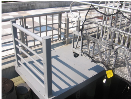
Park design and rules do not allow gangways of homeported vessels to rest on the walkway of the pier, so vessels are obliged to create structures that keep their gangways outboard of the fence. This cantilevered platform was designed and fabricated by ship LILAC, an additional cost.
