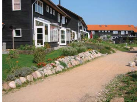
Building Exteriors and Landscape
