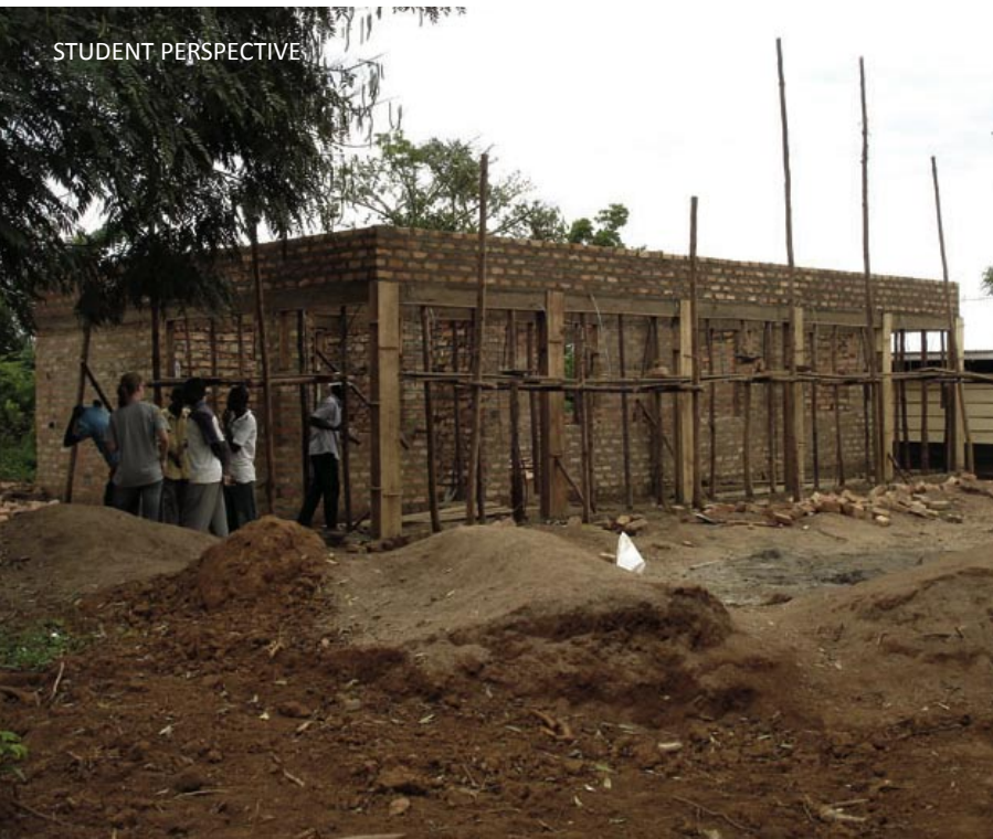
the library in progress
