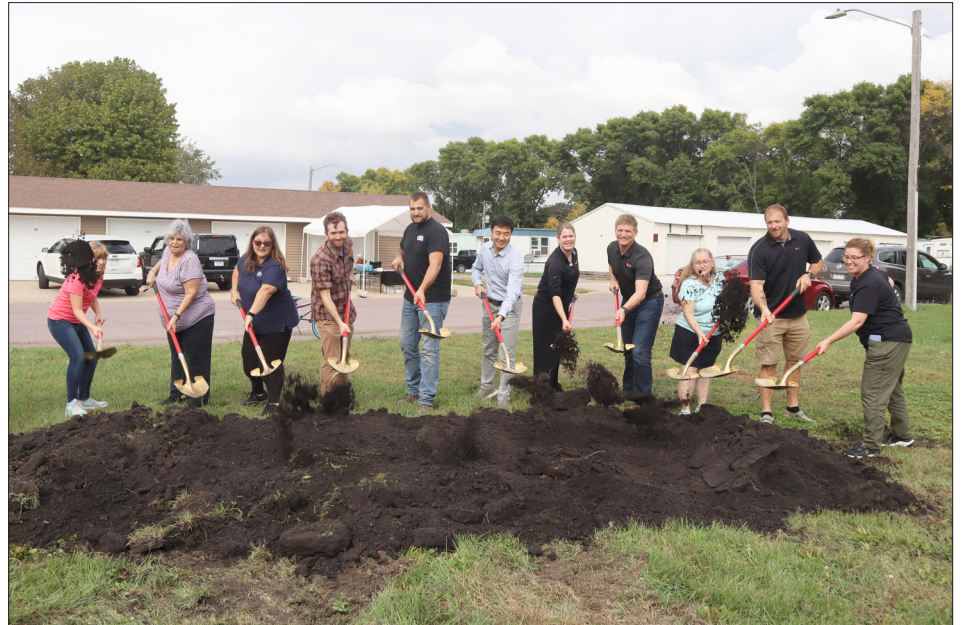
Madelia Mobile Village Cooperative members and project partners break ground on the Cooperative's storm shelter project on September 27, 2023.
