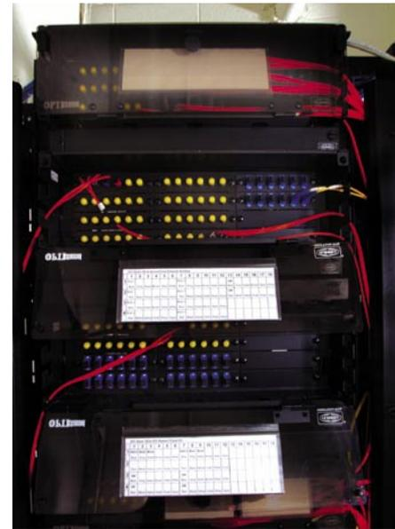
**Front view of local and wide area fiber patch panels in the communications room of the Central Station building**
