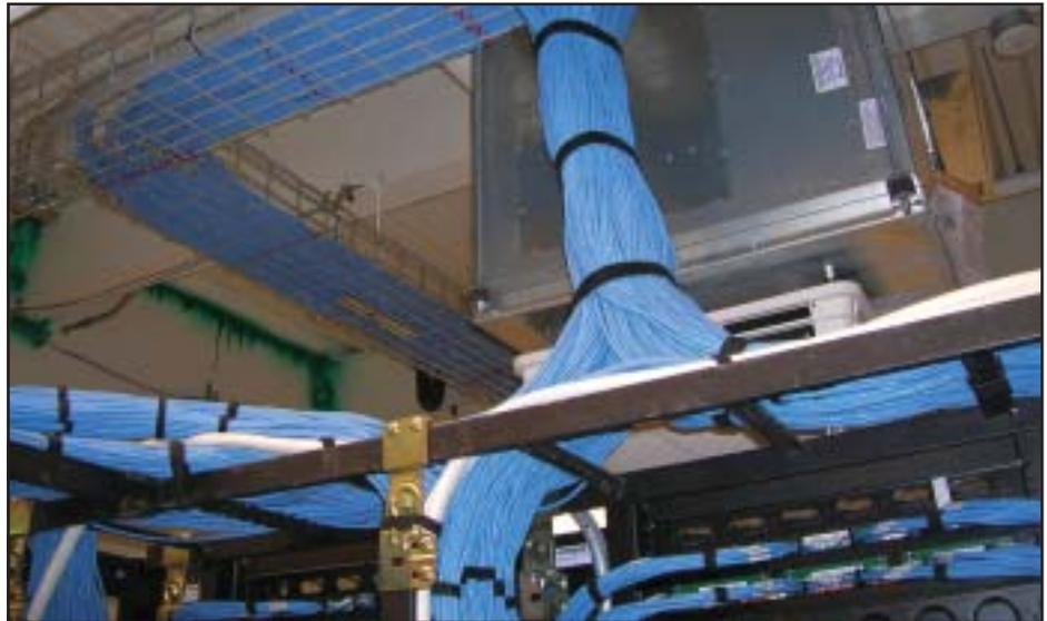
*Any of these Cat6 cables that route back to the panels in the communications room could be used for transmitting video and audio signals between classrooms or back to the video distribution headend equipment.*
