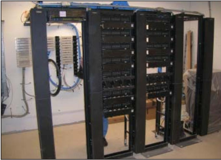
*The racks in the main communications room provide a central location for Cat6 cables and fiberoptic cables installed throughout the building.*
