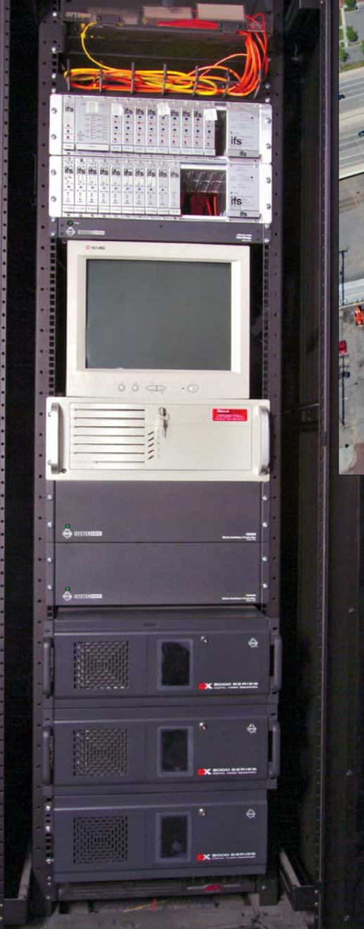
At left, a security office cabinet contains fiber patch panels, fiber to coax transceivers, access control/intrusion detection computer, switching matrix and digital video recorders. Above, a new Central Station complex for the Grand Rapids, Mich., Interurban Transit Partnership is protected thanks to an integrated security design.
