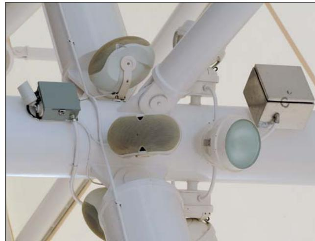
Above, infrastructure is an important element of the security and communications design at the Grand Rapids bus station. Columns on the Central Station platform hold lighting, audio and security video cameras with the latter attached to a pullbox allowing all cables to route through the structural column.
