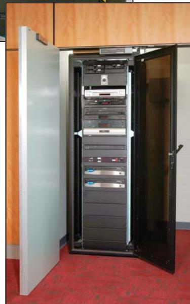
(Top) The communications rack inside the multi-use building incorporates the volume control and AM/FM tuner and CD player connected to the platform and whole building paging system. (Above) This audio-video cabinet is in the side room of the community room.
