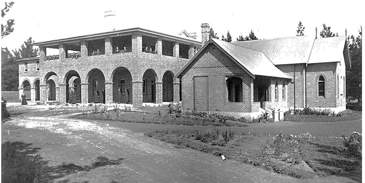
Mittagong: the New Hermitage just after Blessing and Opening. Note novices on verandahs and balconies. Also the newly planted garden. How things have changed.
