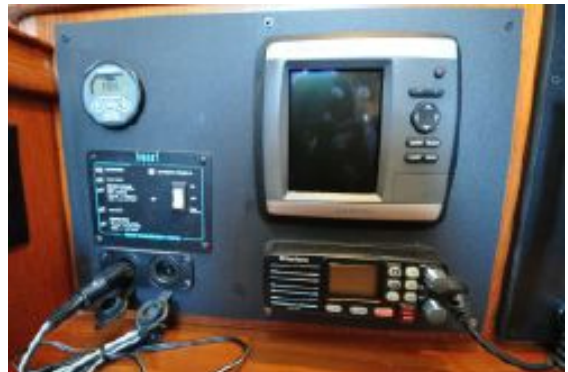
> nav station electronics
