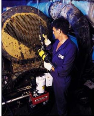
The steel tube sheet within the condenser can also be severely corroded. In extreme cases the steel can become so pitted around the copper condenser tubes that water can leak into the refrigerant system. This is a major and costly repair that requires the chiller to be out of service for long periods of time.
