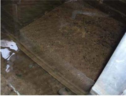
East-West cooling tower, showing sump strainer covered in debris and scale.
