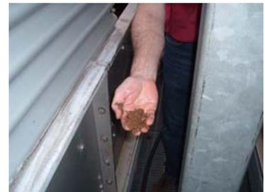
Rust and corrosion particles as well as calcium buildup on the spray and distribution nozzles will reduce water flow. This condition contributes to
