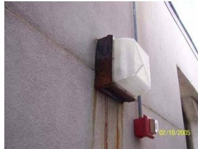
North-South cooling tower, showing tower overspray creating rust and corrosion.
