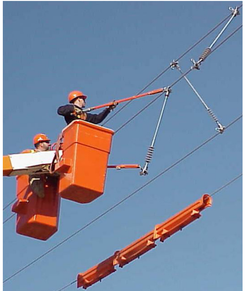
InterPhase Spacer installation using Hot Line Tools
