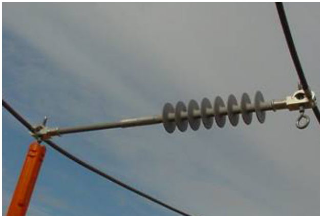
InterPhase Spacer installation using Hot Line Tools
