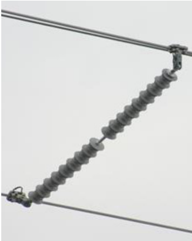
Transmission Line InterPhase Spacer
