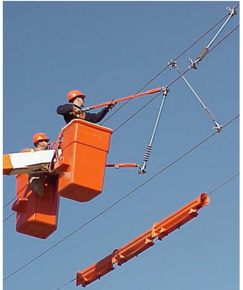
InterPhase Spacer installation using Hot Line Tools
