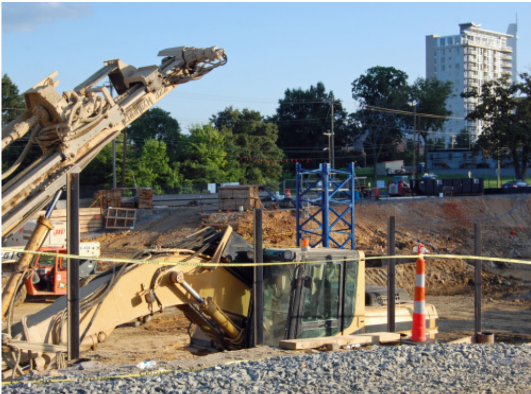
( http://centercity2020.files.wordpress.com/2009/10/3838056675_ec6ab1a02c_o.jpg ) UNC Charlotte's Uptown Campus under construction
